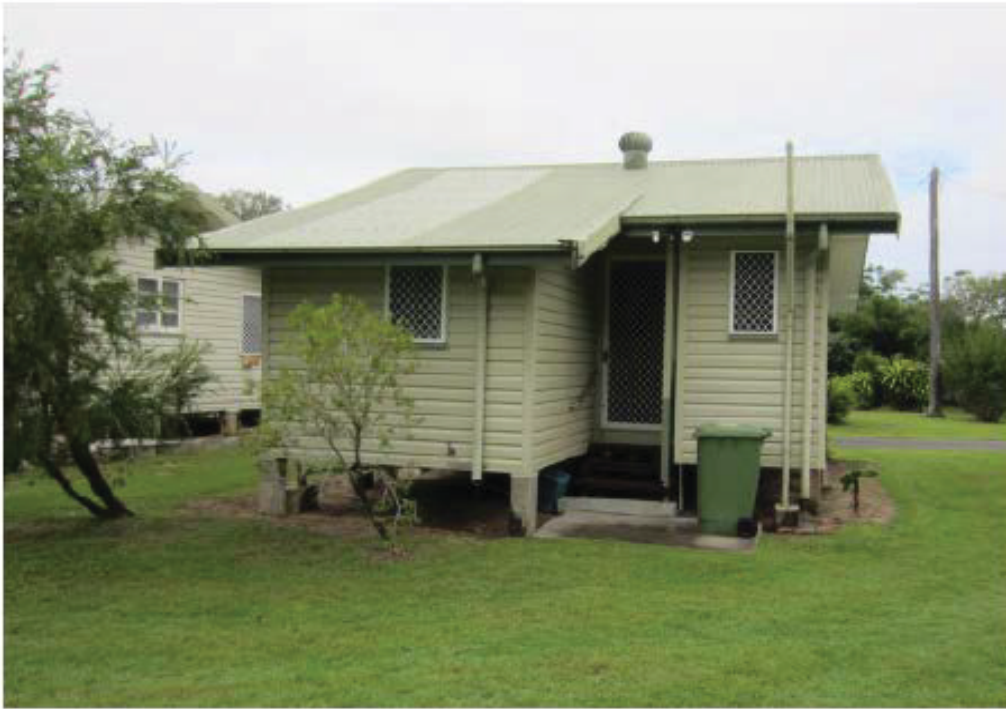
Figure 4: Rear view of one of the cottages (Source: EHP site visit 06/05/13)
