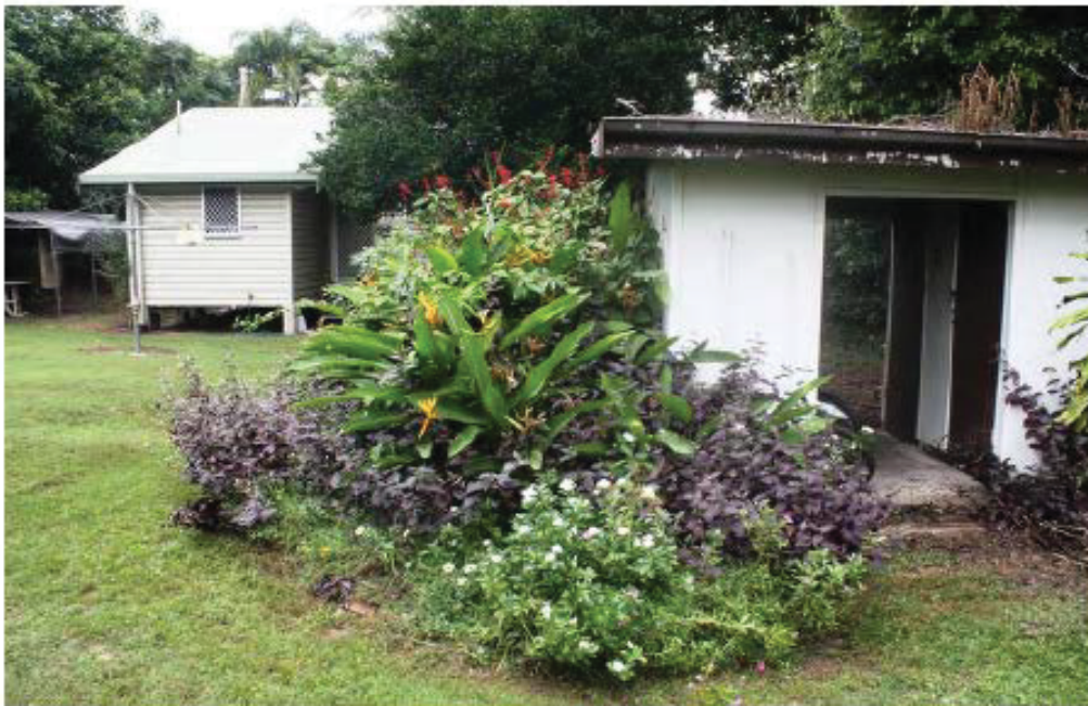
Figure 5: View towards Cottage 8 and Laundry Block 2 at the rear of the site (Source: EHP site visit 06/05/13)
