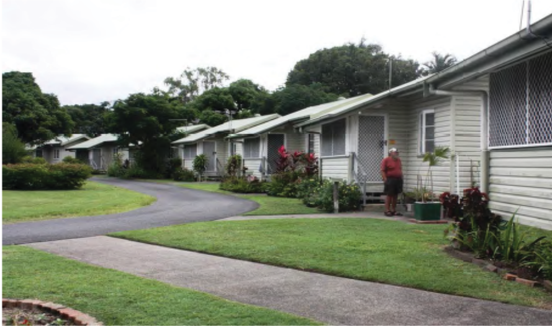
Figure 1: View along the pensioners' cottages (Source: EHP site visit 08/05/13)
