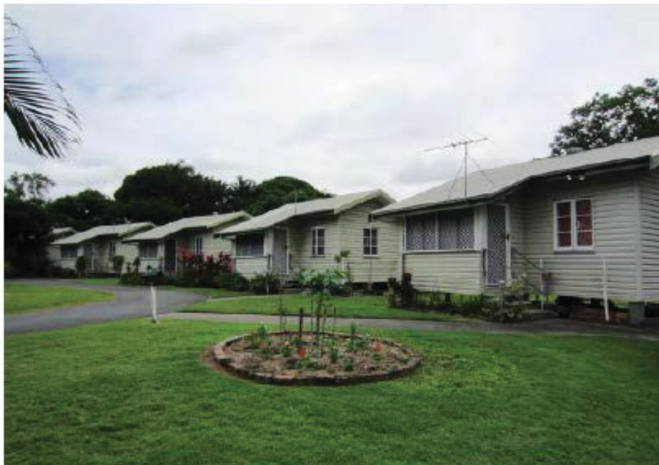
Figure 3: View of the cottages from the front lawn (Source: EHP site visit 06/05/13)
