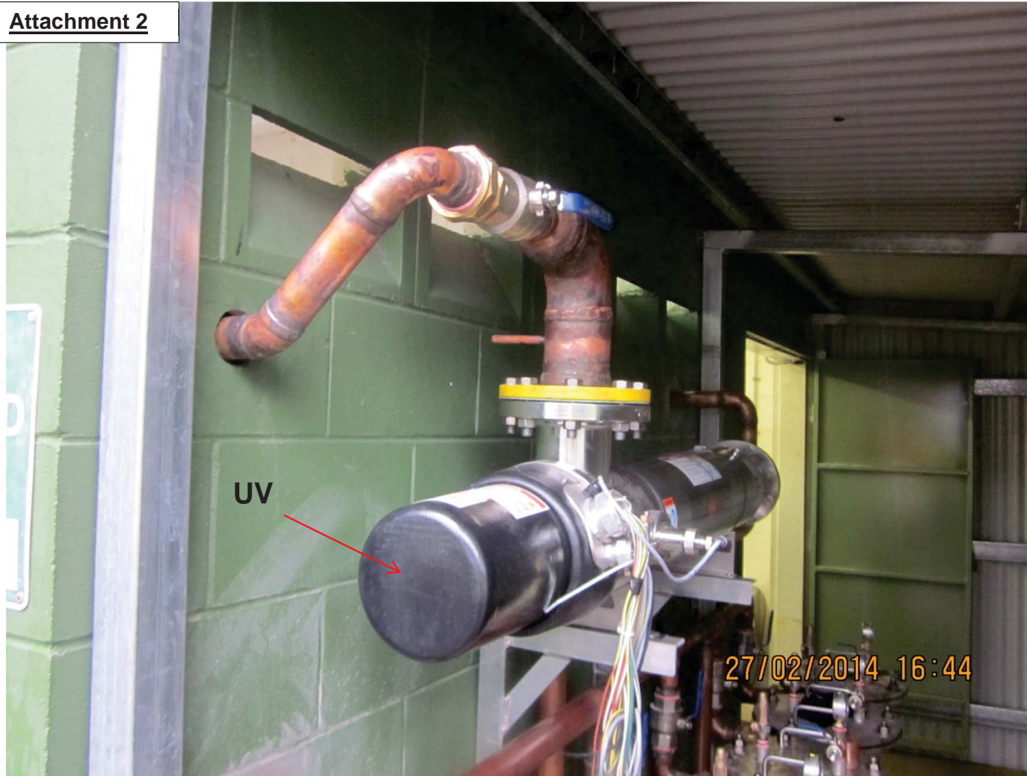
Figure 1: UV installation at Orchid Valley
