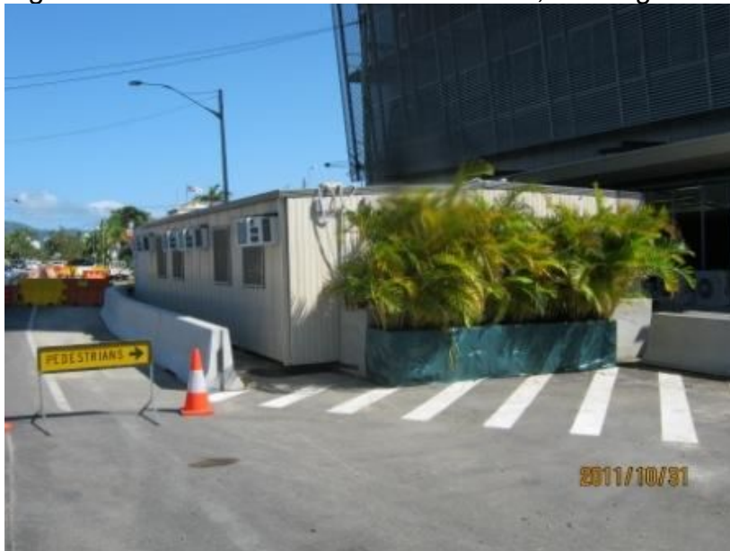
Figure 2 - North End of Site Offices
