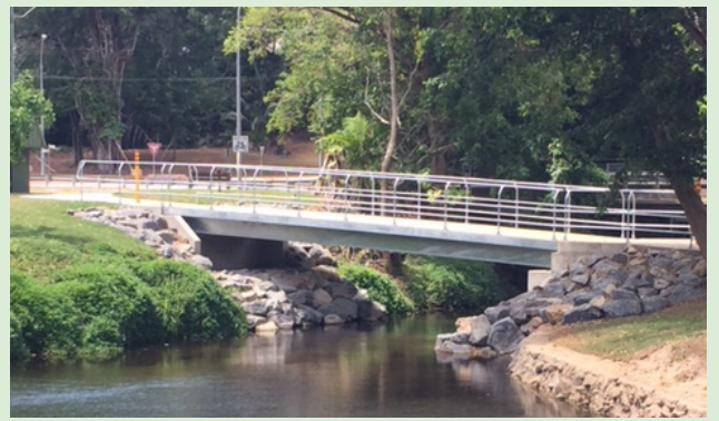
The cycleway enables riders to safely cross the bridge near Ryan Weare Park
