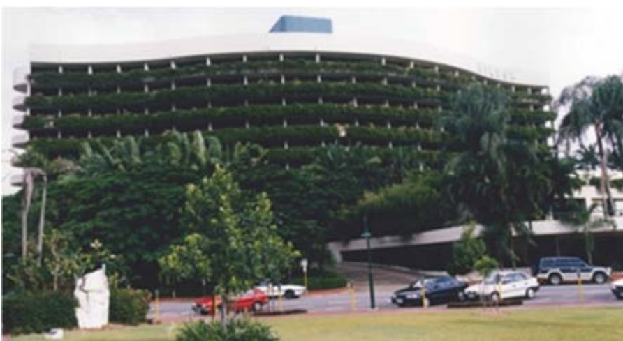
Figure SC6.16.3.7.e – Example of vertical landscaping – Cairns Hilton
