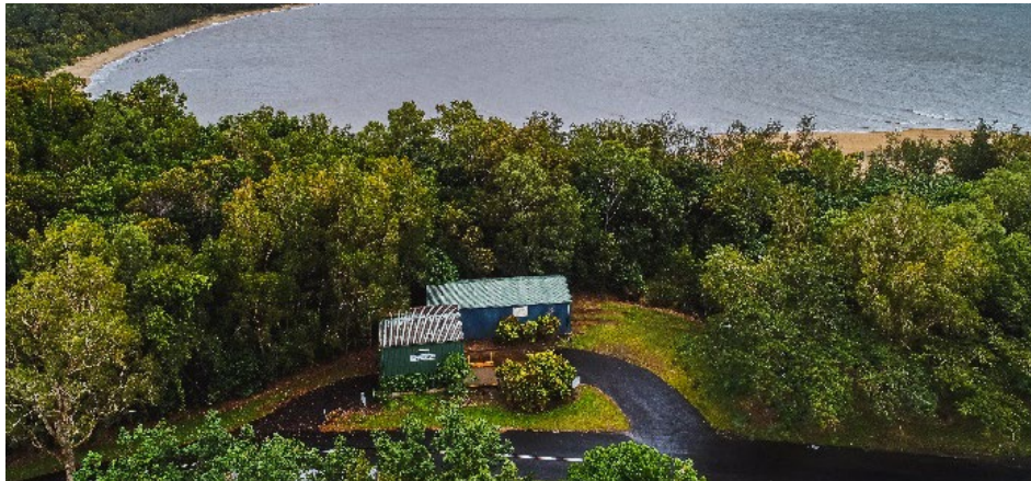
Bramston Beach Drop Bin aerial images.
