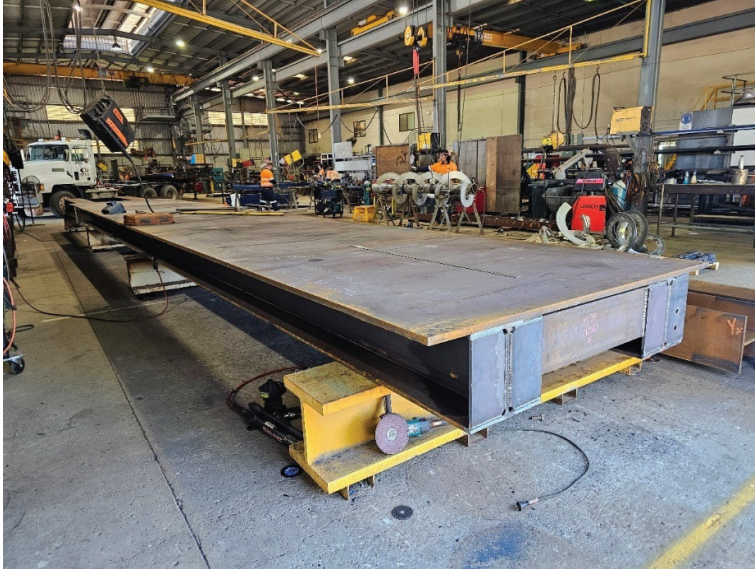
Segment of the steel bridge under construction at Dawsons Engineering.
